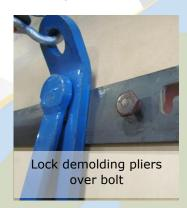
4. Open the docks at either end of the wall section being stripped but do not open those holding the panels being stripped together. Before hoisting, place the mobile chains holding demolding pliers vertically over pliers to balance load. Slowly hoist panels with a slight angle away from the wall keeping load as balanced as possible.
